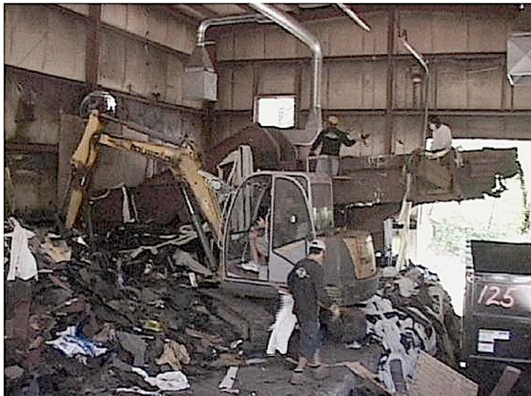
Picture 13 - Grapple Crane Servicing Indoor Loads of Mixed Roofing Materials (Together with Floor Picker Coupled With Elevated Sort Line)
